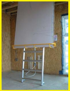
Safety Platforms are delighted to launch their new "Easy-Load" bracket which removes the need for carrying heavy plasterboard sheets up stairwells by allowing sheets to be passed up through a letterbox in the floor. Up to five 33kg sheets can be loaded onto the bracket, the operatives then walk to the upper floor, remove the sheets and stack them ready for use.
