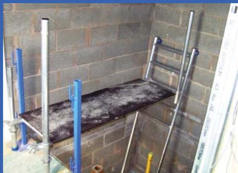
**Guardrail posts fitted**
