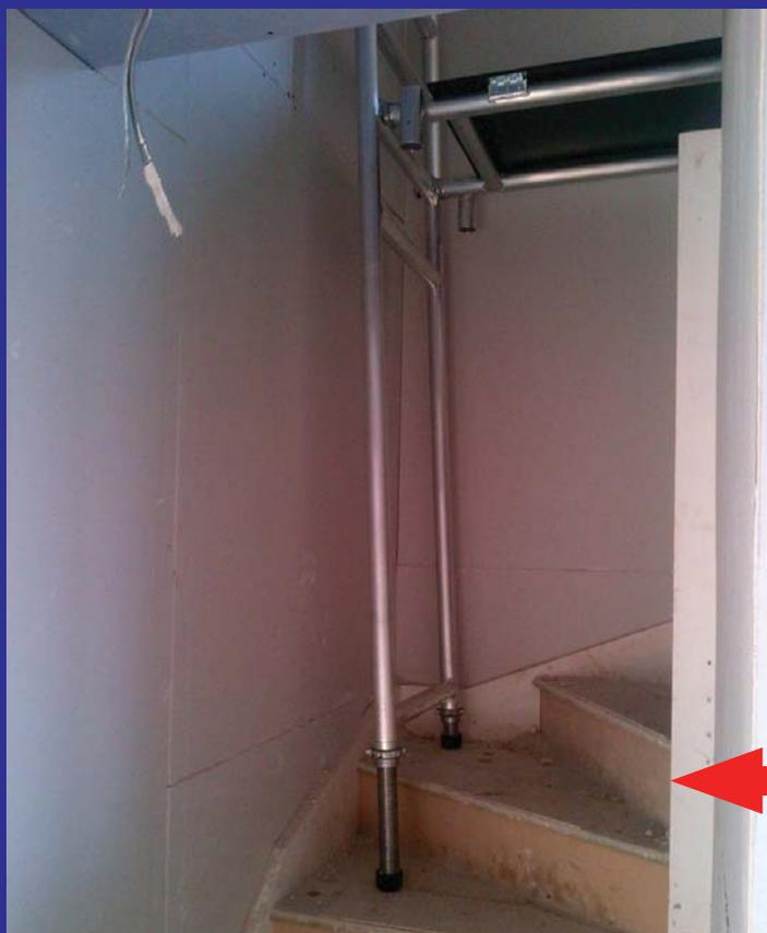
Stairsafe frame supports kitewinder platform at lower end of stairs
