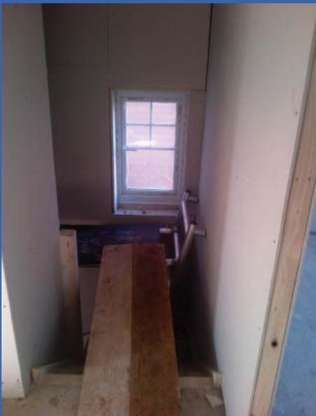
Where required an additional Stairsafe platform or scaffold boards (as shown) can be used to provide access onto the platform from the top of the stairs.
