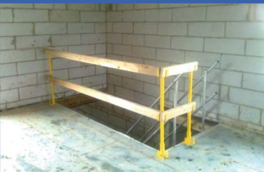
**Stairsafe when used in conjunction with suitable edge protection addresses all stairwell safety issues**
