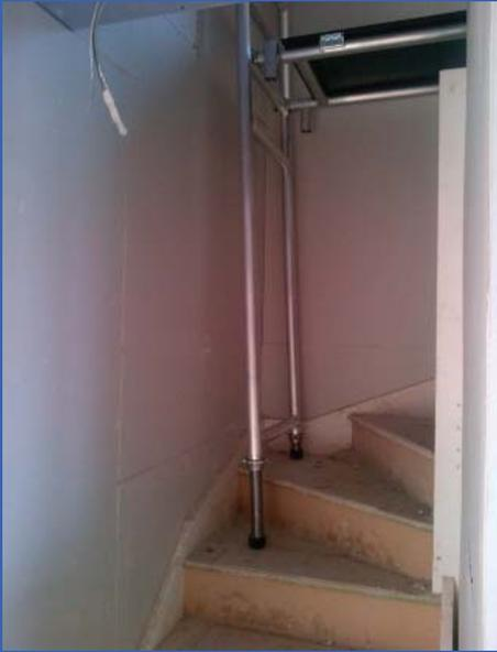
1. Position Stairsafe ladder frame at lower end of stairs
